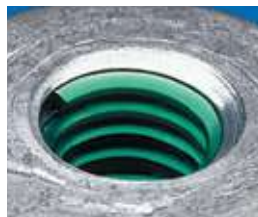
Repaired thread
